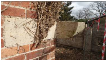
Plate 6 Stone corbel at southeast corner of sawpit
