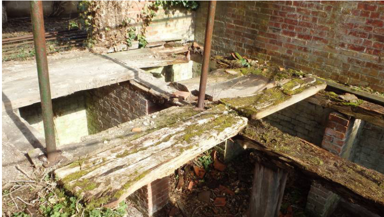
Plate 25 Timber planks and joists of sawpit, looking northeast
