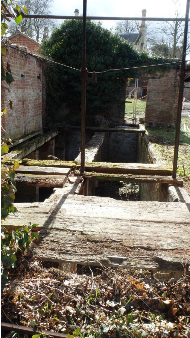
Plate 22 General view of sawpit interior from north
