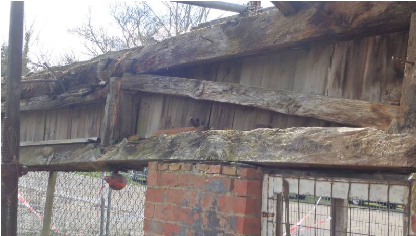
Plate 19 Timber structure of west wall of sawpit viewed internally
