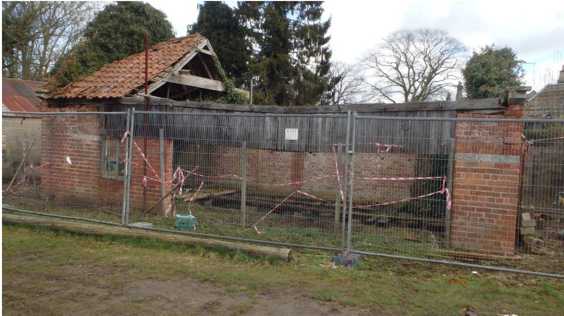
Plate 15 West elevation of the sawpit
