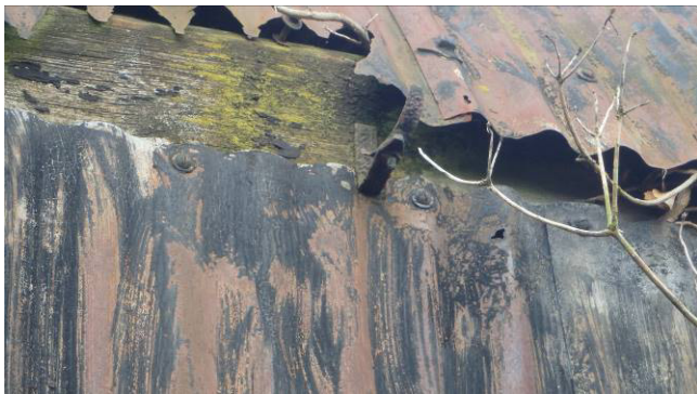
Plate 41 Iron guttering fixing attached to Dutch barn
