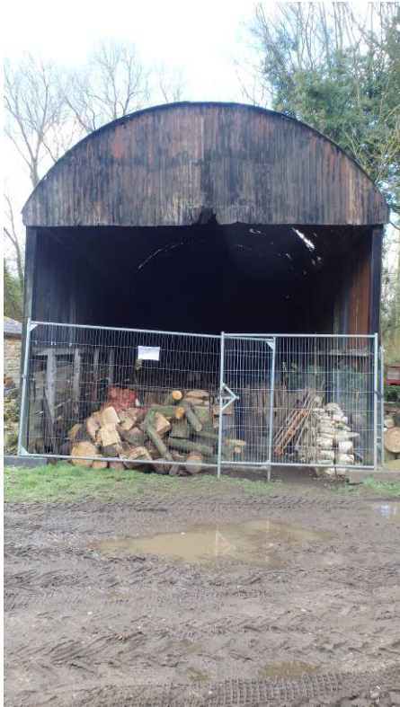
Plate 32 East elevation of Dutch barn
