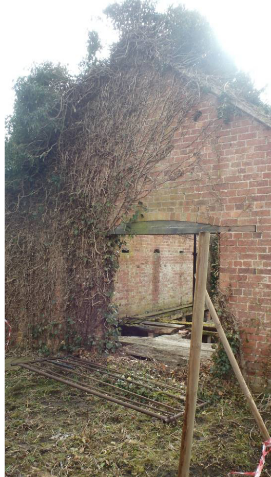
Plate 14 North gable of sawpit, looking southeast
