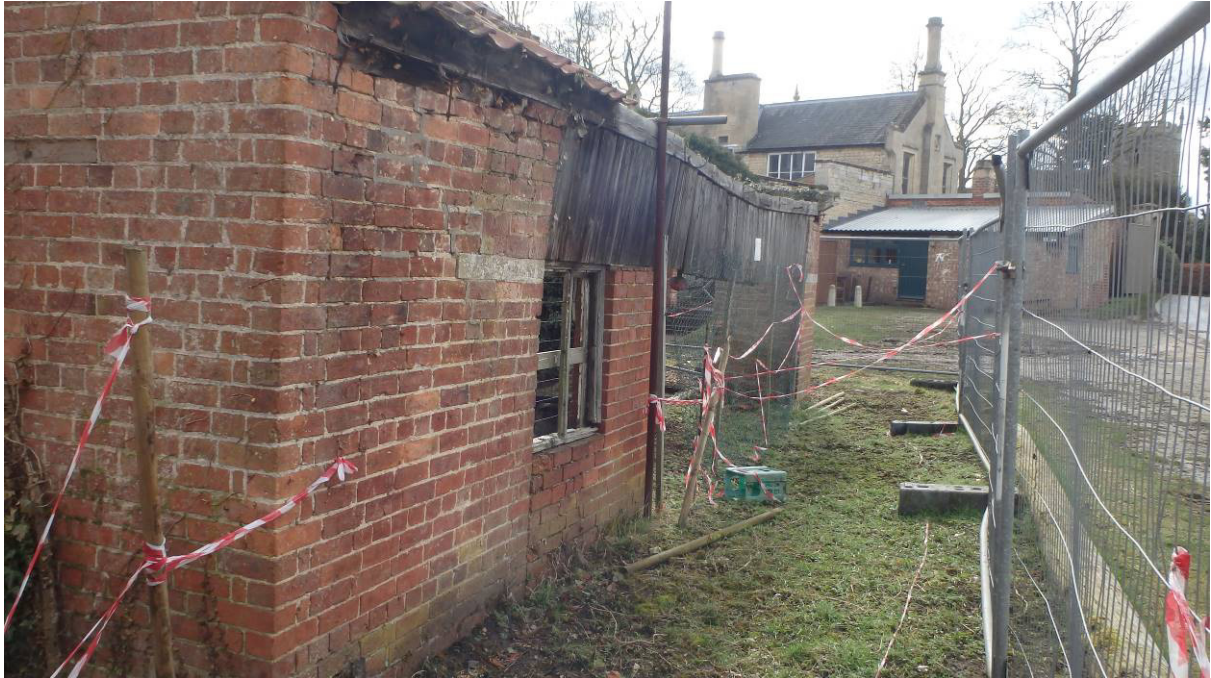
Plate 17 West elevation of sawpit showing brick infill with inserted window
