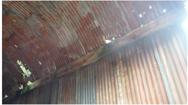
Plate 39 Detail of timber in north wall of Dutch barn frame
