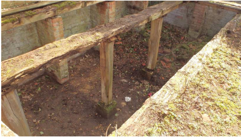
Plate 23 Sawpit, looking southeast
