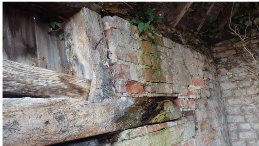
Plate 20 Detail of brick and timber structure of west sawpit wall
