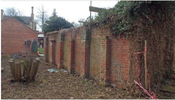
Plate 10 East elevation of sawpit, looking southwest
