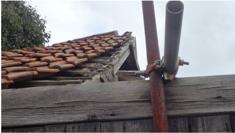
Plate 28 Detail of sawpit roof structure externally
