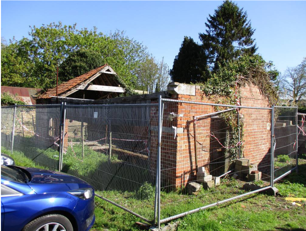
Plate 1 General view of the sawpit from southwest
