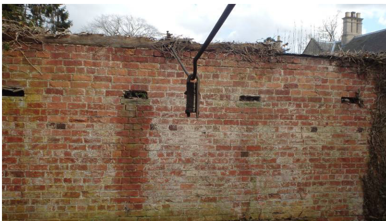
Plate 27 Iron bar spanning sawpit with iron device attached
