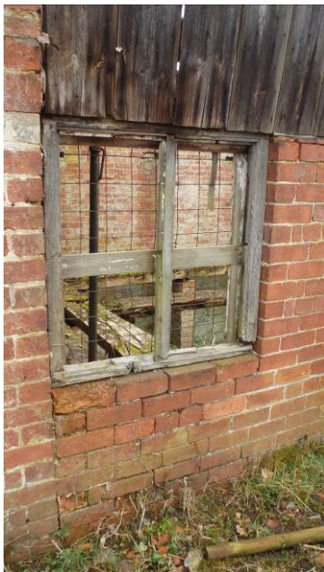
Plate 18 West elevation of sawpit, detail of inserted brickwork and window
