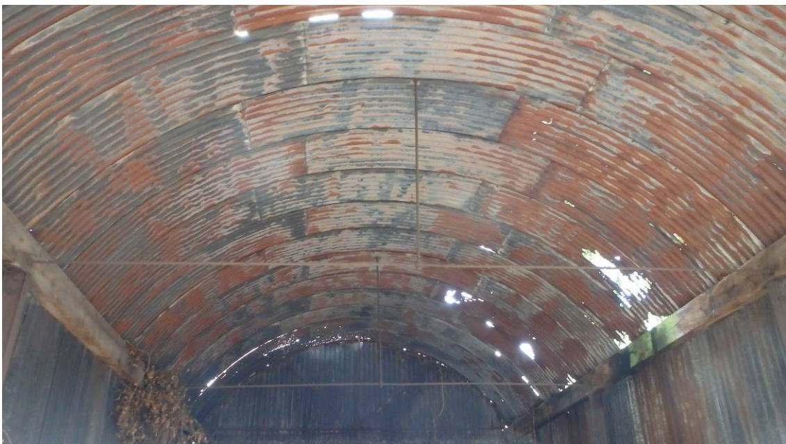
Plate 38 Roof structure of Dutch barn
