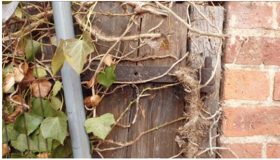
Plate 5 Iron hinge and pintle of south door of sawpit
