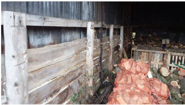
Plate 40 Detail of wood infill in north wall of Dutch barn
