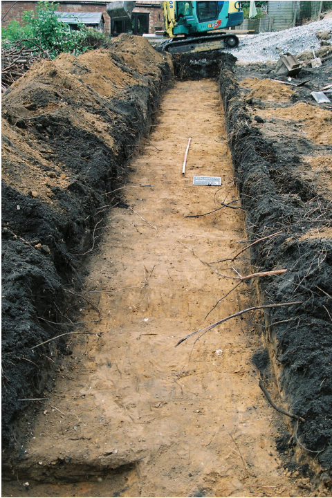
Plate 4 Trench view, looking south
