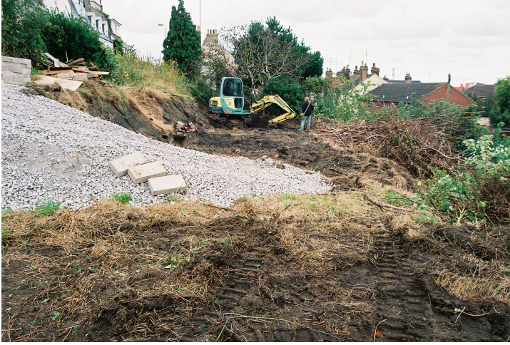
Plate 1 Level area of site, looking north
