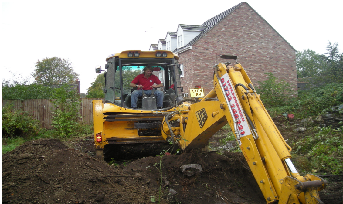
Plate 2 Work in progress
