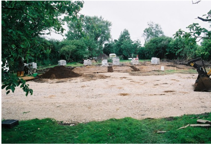
Plate 1 North facing view across site showing completed house footings
