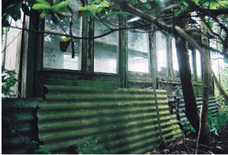
Plate 7 West facing view summer house showing former railway carriage panel
