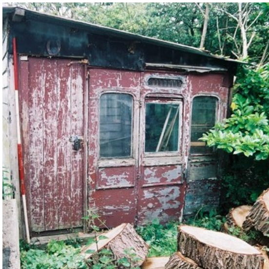
Plate 6 North facing view summer house showing former railway carriage panel
