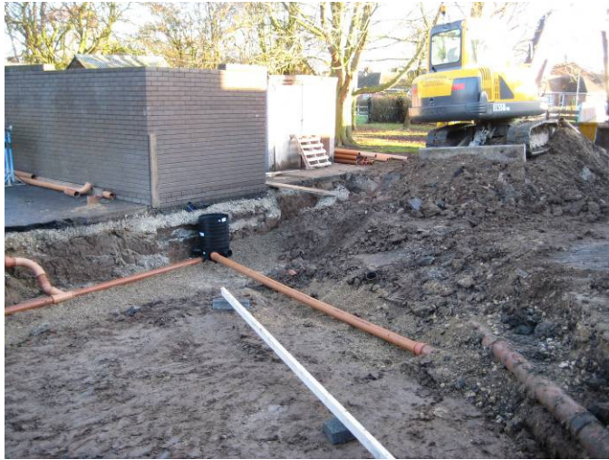
Plate 1 East facing view across development area showing work in progress
