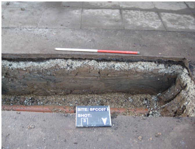
Plate 2 South facing view Section 1
