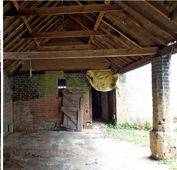
Plate 13 Inside the cartshed looking northeast to the stable
