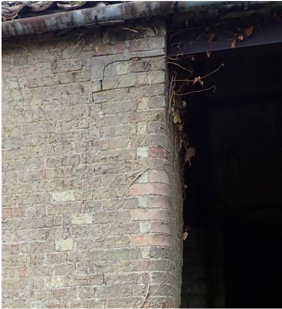
Plate 15 (left). Detail of the bullnose bricks at the northern end of the cattle accommodation
