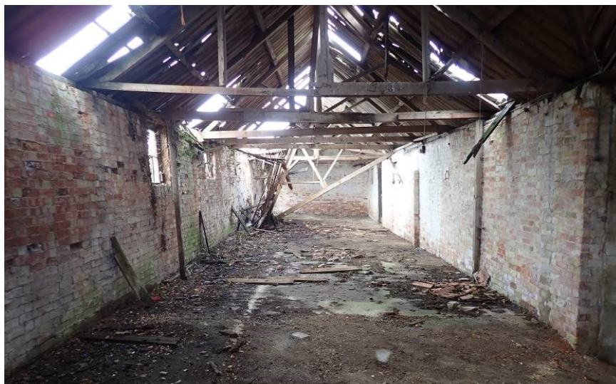
Plate 28 . Room 5, cattle accommodation, looking southwest
