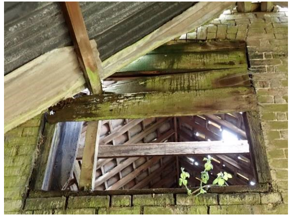
Plate 8 (above). The original gable end and pitching door in the southeast elevation of the threshing barn
