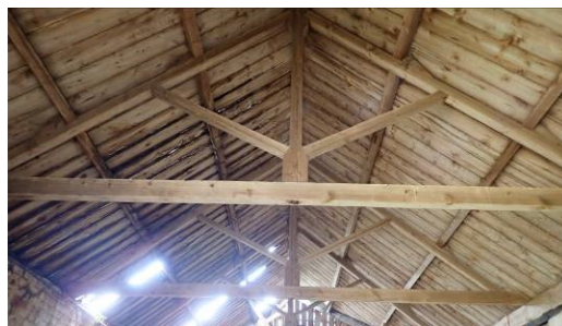
Plate 27 (below). Detail of the king post roof trusses in Room 4
