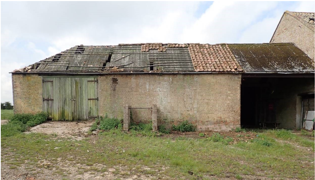
Plate 14 The northeast elevation of the cattle accommodation
