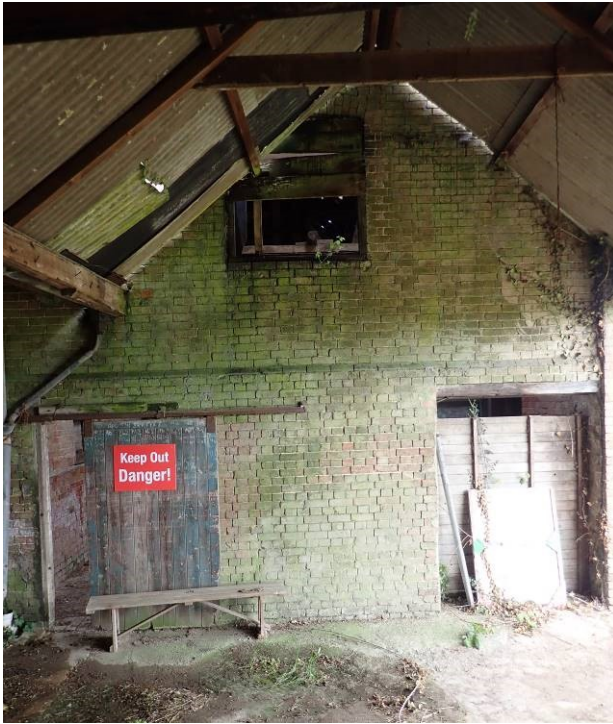
Plate 8 (above). The original gable end and pitching door in the southeast elevation of the threshing barn
