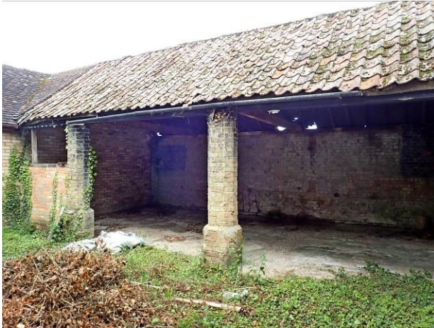
Plate 12 The southeast elevation of the cartshed, looking northwest
