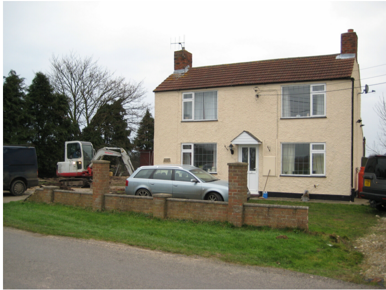
Plate 1 – View of Lynton Cottage with work in progress, looking east
