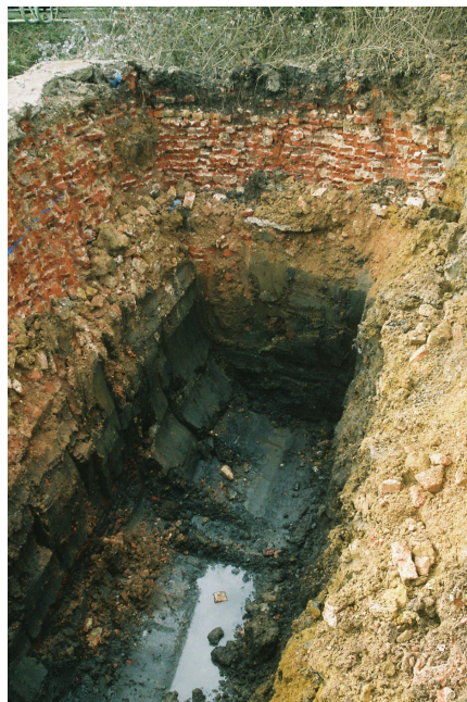
Plate 3 – Northern bridge pier pit with bricks of former bridge, looking southwest
