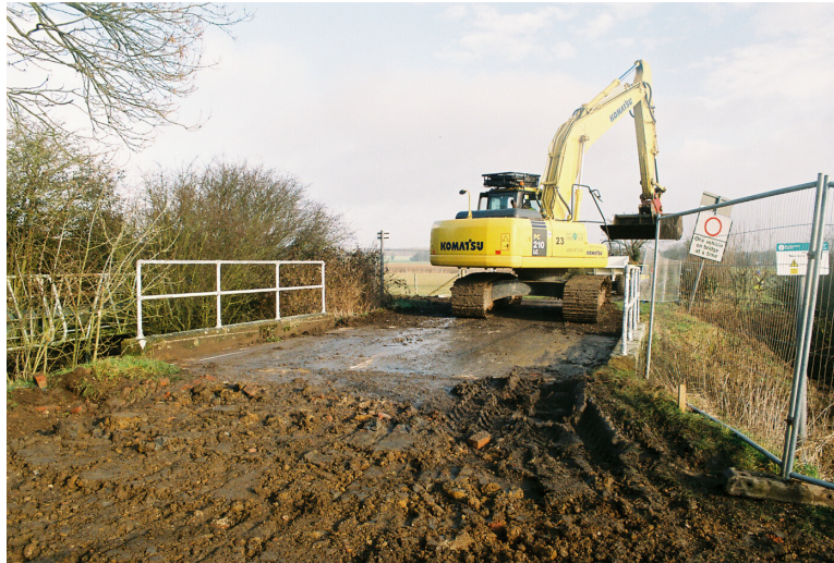
Plate 1 – General view showing West Lane Bridge, looking north
