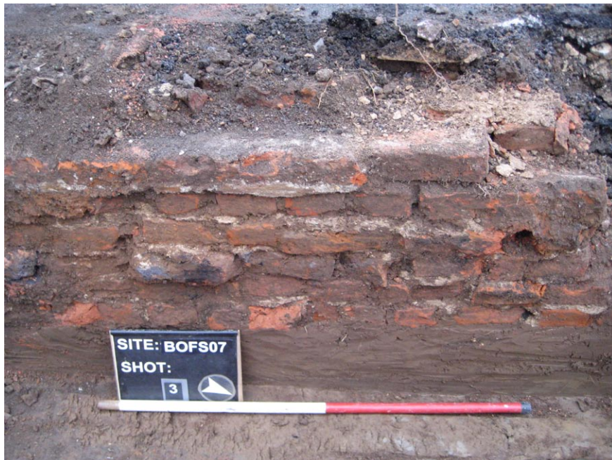
Plate 2 Section 2, showing wall footing (003), looking WSW
