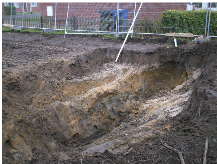
Plate 3 – Plot 5 during excavation, looking northwest
