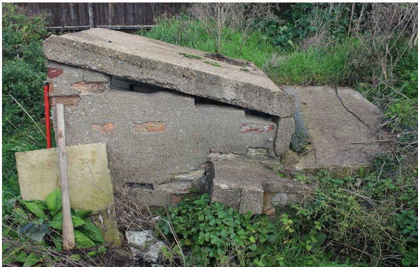
Plate 2. The south elevation of the shelter entrance
