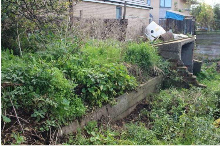
Plate 3. Oblique view of the shelter looking southeast
