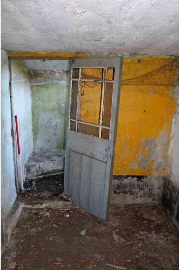
Plate 6. Internal view of the shelter, looking south
