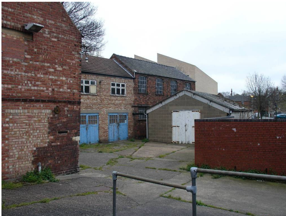
Plate 4: Yards to rear of 29-31 The Strait, looking east
