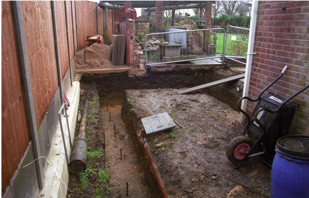
Plate 1 – View of the extension footings, looking southeast
