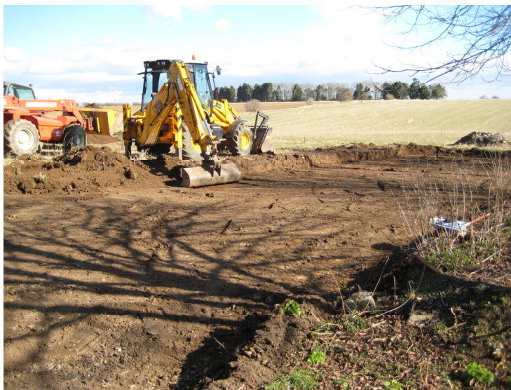
Plate 2 – Stripping off the access road, looking west
