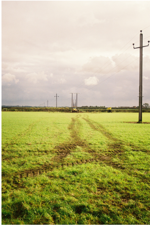
Plate 1 – General view along the length of the works, looking east
