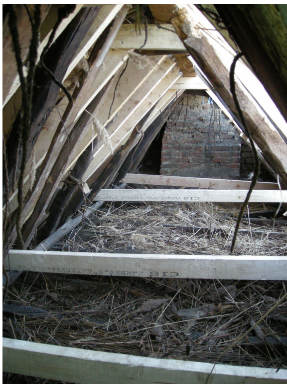
Plate 6 – View showing roof layout with modern timber-framing
