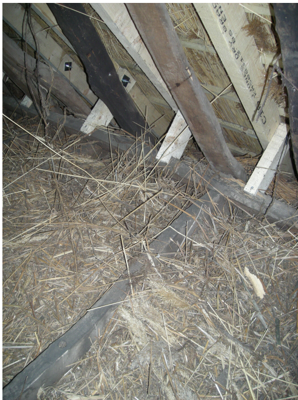
Plate 7 – Detail showing collar and purlin
