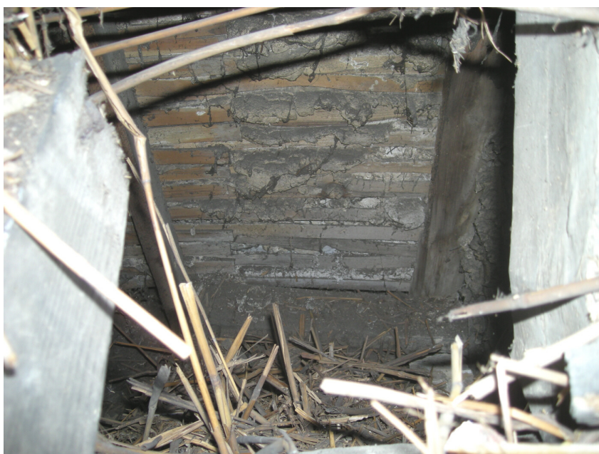
Plate 8 – View showing lathe and plaster wall set back from external face
