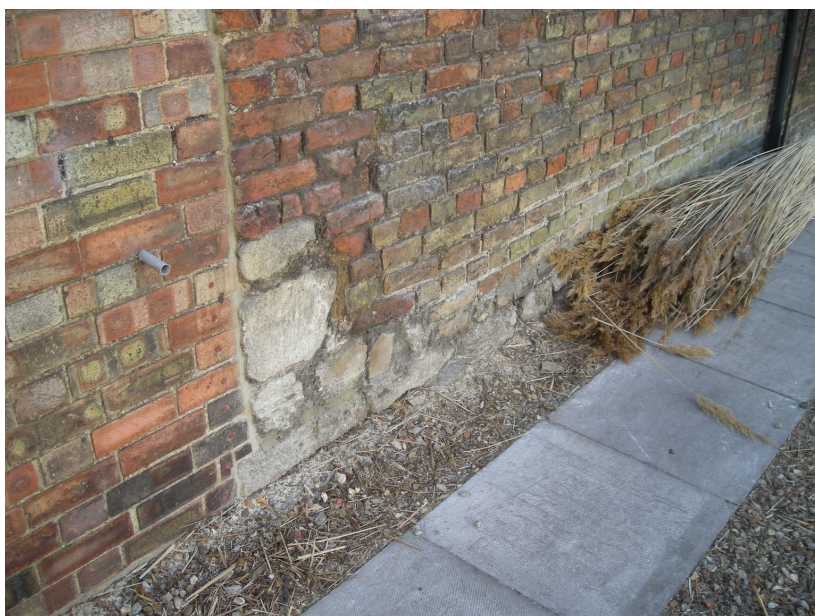
Plate 9 – Stone foundations along north side of the cottage
