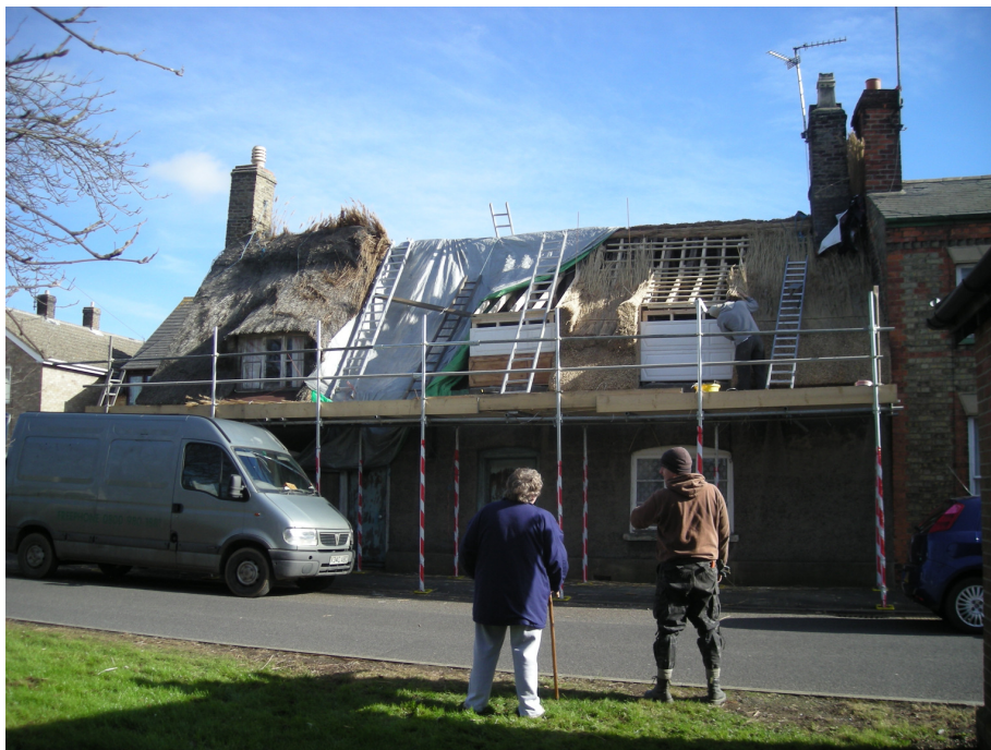
Plate 4 – 45 North Street showing work in progress, looking east
