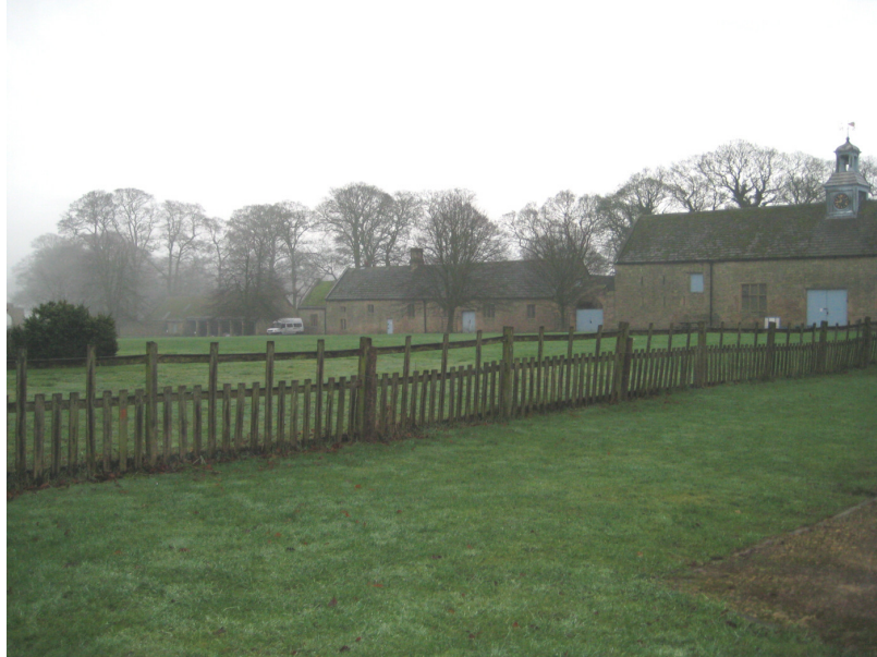
Plate 1 – View of the south range of the Stable Yard, looking southeast
