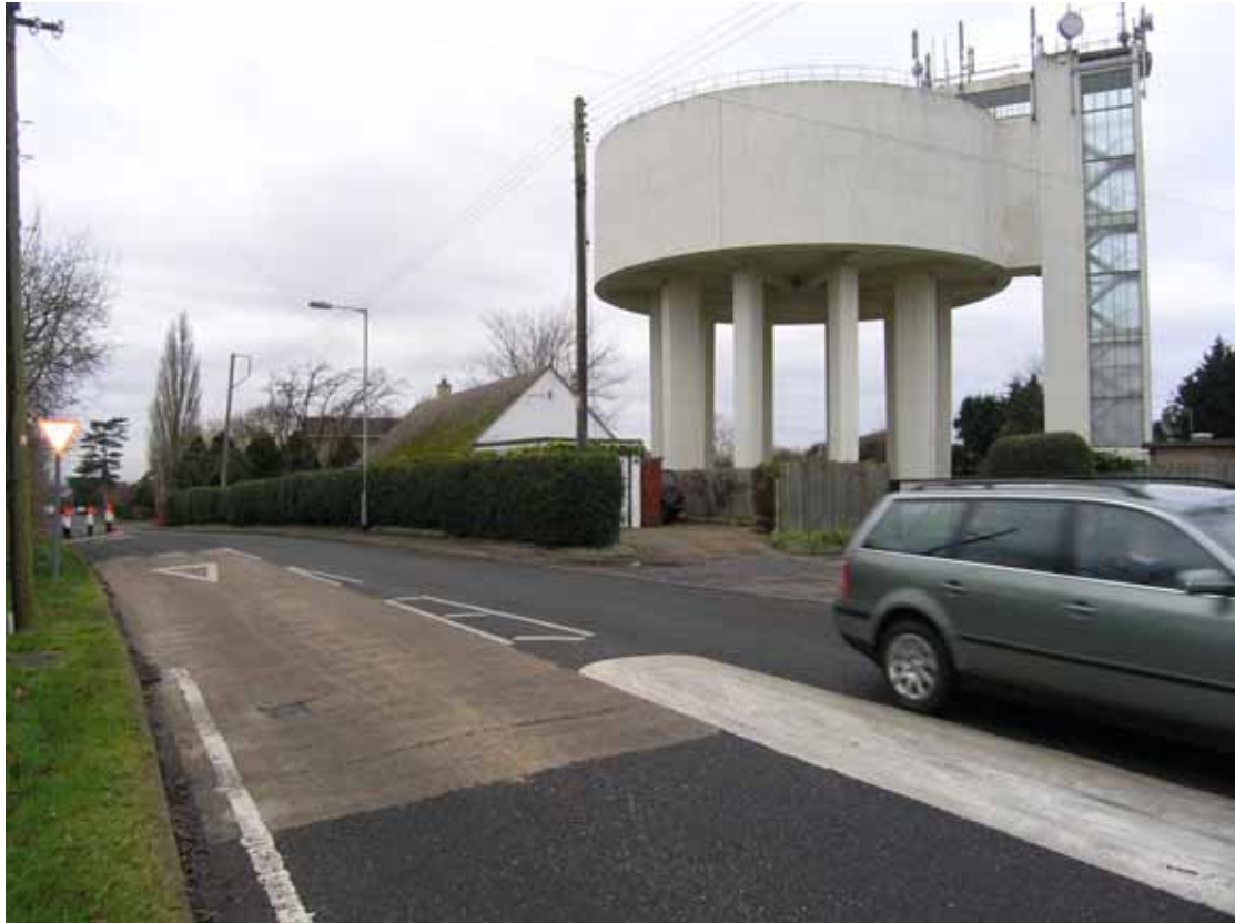
Plate 1 View at southern end of pipeline route, showing water tower at Haddenham, looking northwest
