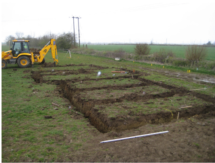
Plate 1 Southwest facing view across development showing completed groundworks
