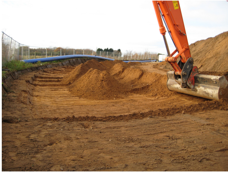
Plate 1 – View showing the stripping of the site, looking northwest
