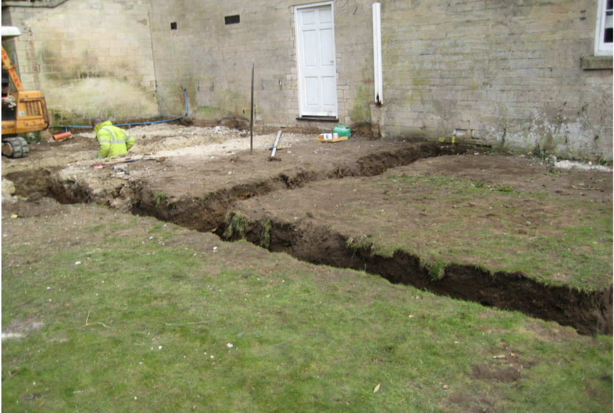
Plate 3 – General view of footings looking northeast
