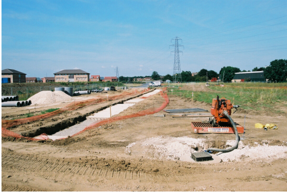
Plate 1 – View looking over the development site, looking west
