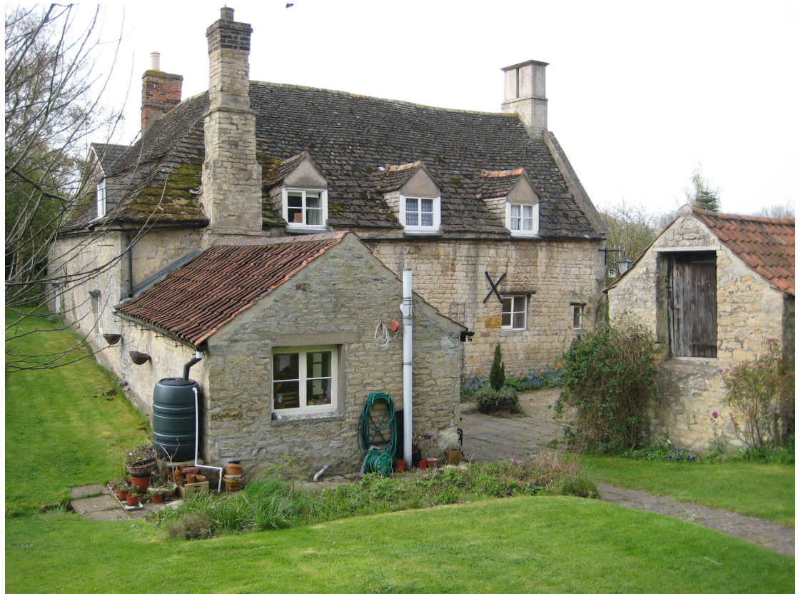
Plate 2 View showing north elevation of kitchen wing to be altered by extension and main building of Bridge Cottage and outbuildings, looking southwest
