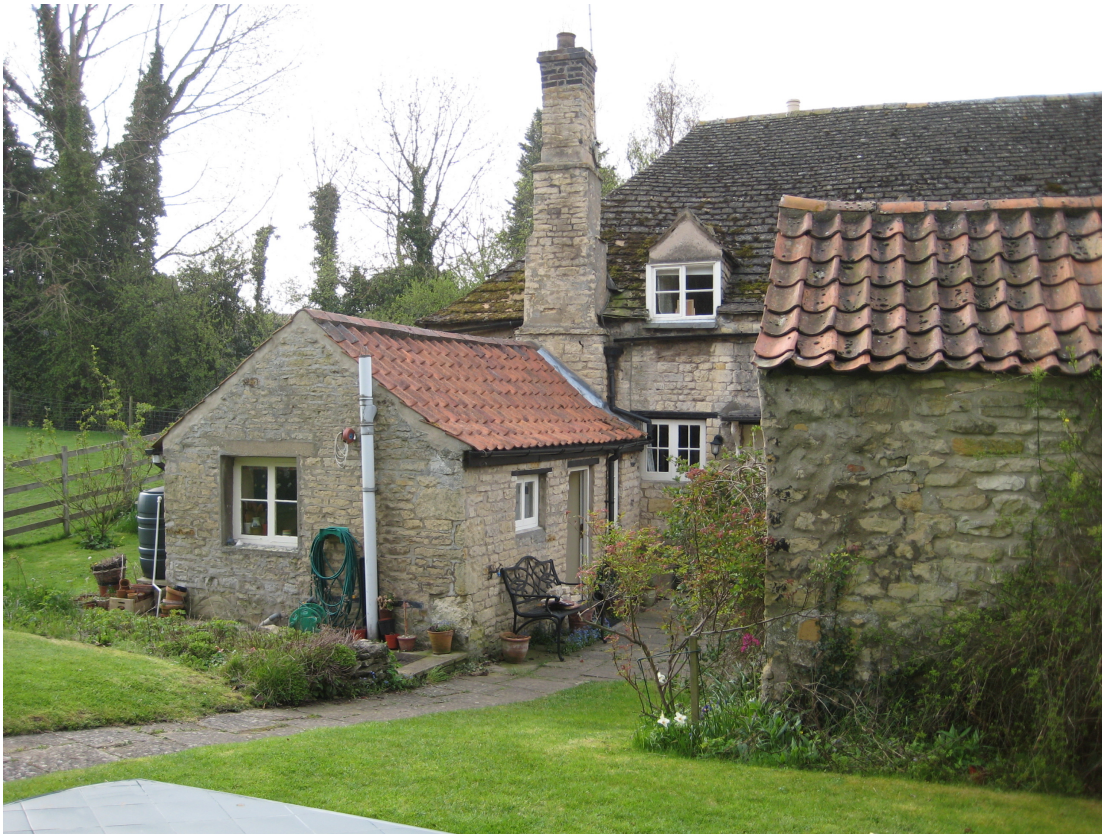
Plate 3 View showing north elevation of kitchen wing to be altered by extension and main building of Bridge Cottage and outbuildings, looking southeast
