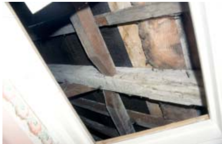
Plate 6 Roof beams within Laburnum Cottage
