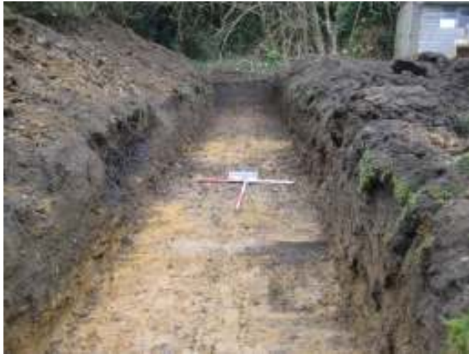
Plate 1 – Trench 1 after cleaning, looking south
