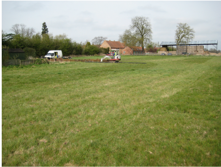
Plate 1 – View of the cable trench, northeast of Swinderby Road, looking northwest
