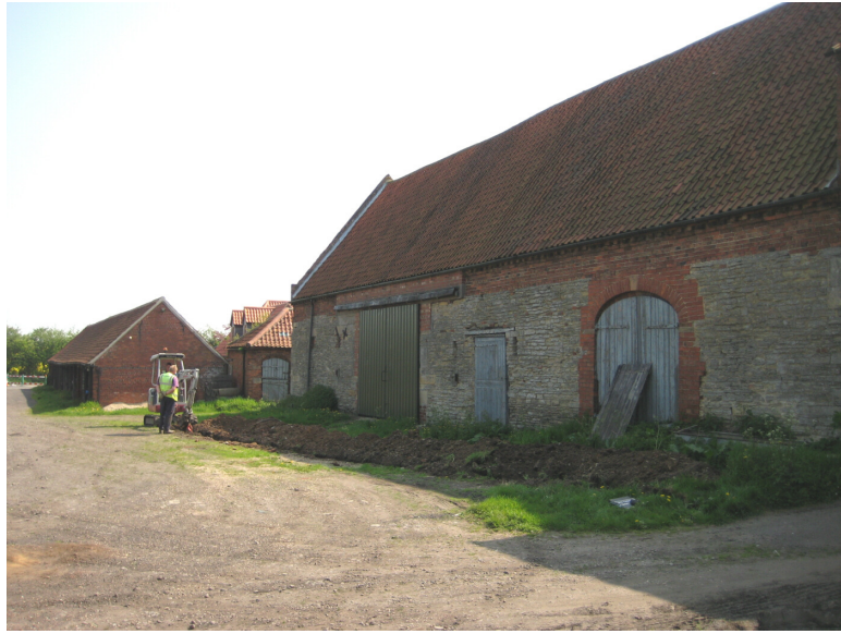
Plate 4 – The cable trench through Eagle Hall Farm, looking east
