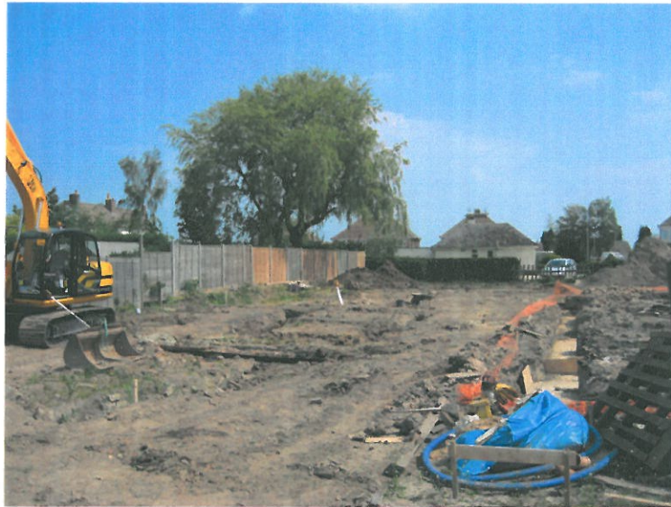
Plate 1 – General view of the site, looking northwest
