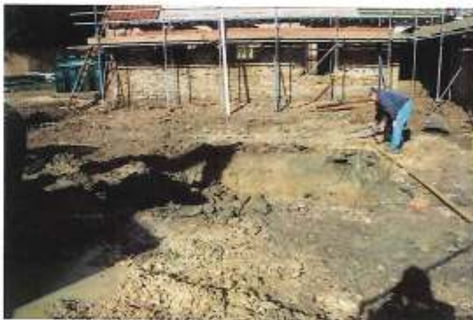
Plate 3 Area 3, looking North West
