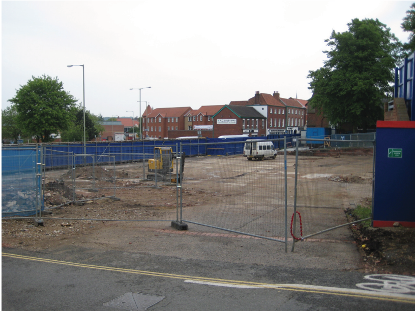
Plate 1 The development site looking east from Wellington Lane
