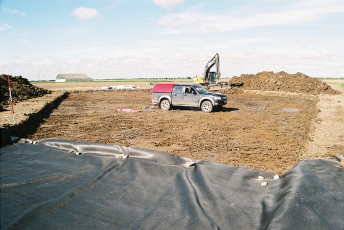
Plate 4 - Area stripped for Turbine 10
