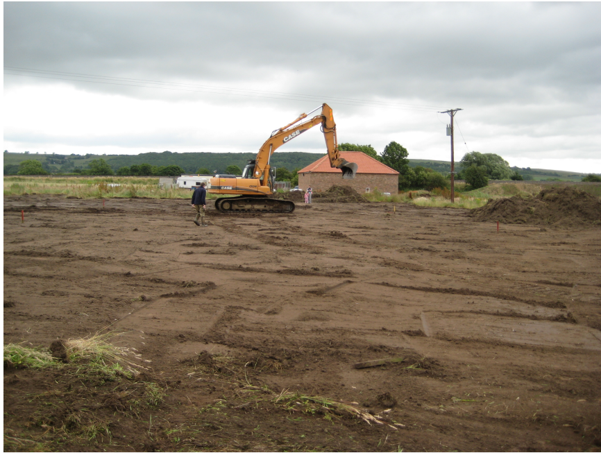
Plate 1 – General view across the stripped area, looking southeast
