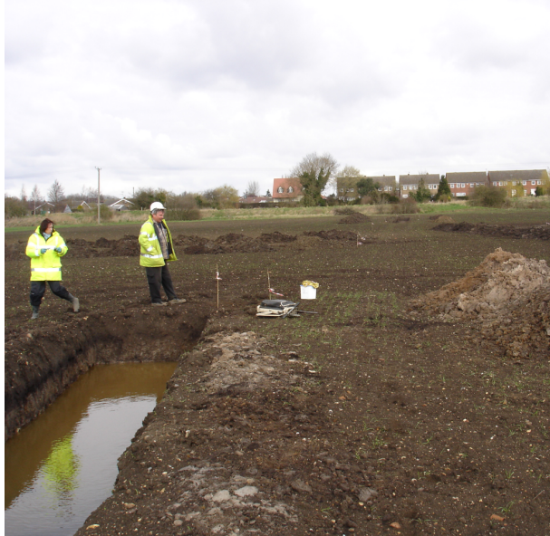
Figure 2. The line of five boreholes is laid out northwards from BH1 just by the white tub. The trench in the foreground is Trench 23 and those in the background Trenches 18 and 10. The land drops 0.4m between BH1 in the foreground and BH3 fifty metres to the north.
