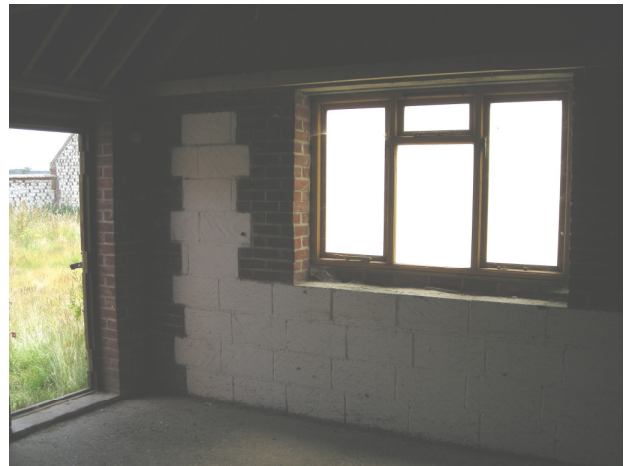
Plate 10 – Modern south wall of Building 2
