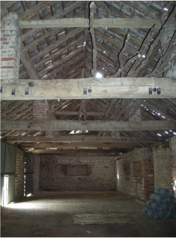
Plate 7 – Threshing barn, roof detail
