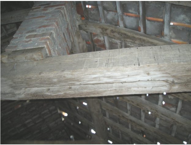
Plate 8 – Threshing barn showing brick pillars supporting principal rafter
