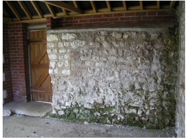
Plate 9 – Building 2, interior view showing modern door and original walling, looking southwest
