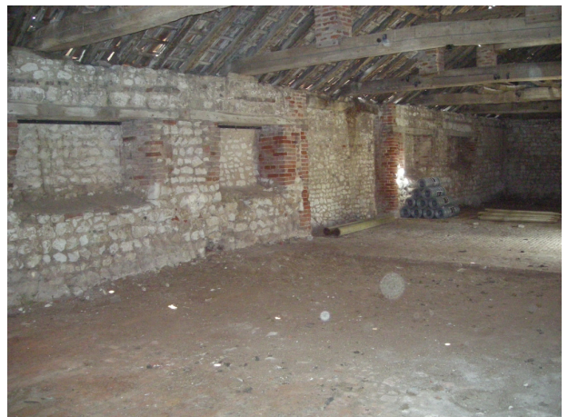
Plate 6 – Interior view of the barn showing the blocked openings on the north wall
