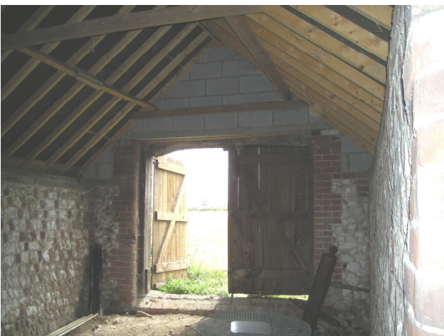
Plate 14 - Interior view of Building 4 showing recent roof
