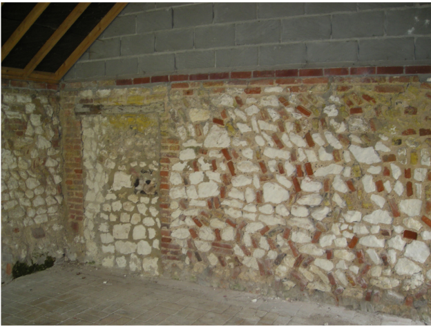
Plate 13 – Building 3, blocked doorway on the north wall
