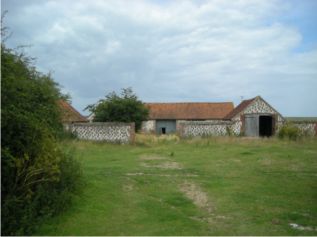
Plate 1 – Marsh Farm, looking north
