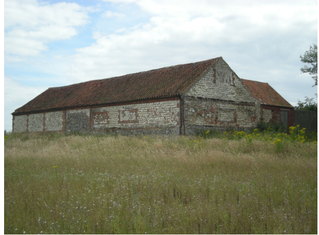
Plate 4 – The north and west elevations showing blocked openings from the northwest
