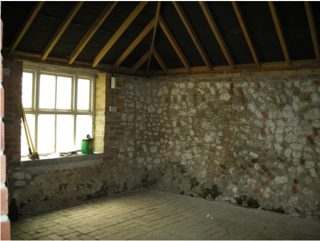
Plate 12 – Interior view of Building 3 showing brick floor
