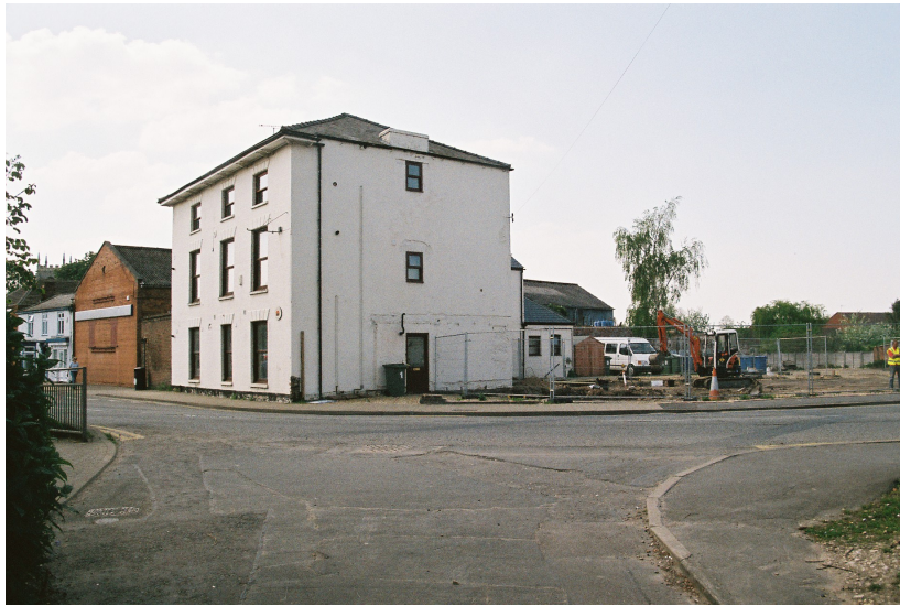
Plate 1 – General view of the development area, looking southwest
