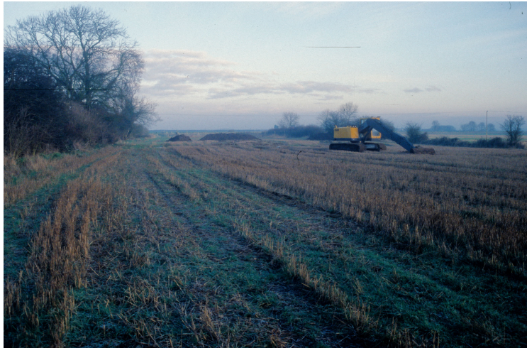
Plate 1 – General view of the site, looking south
