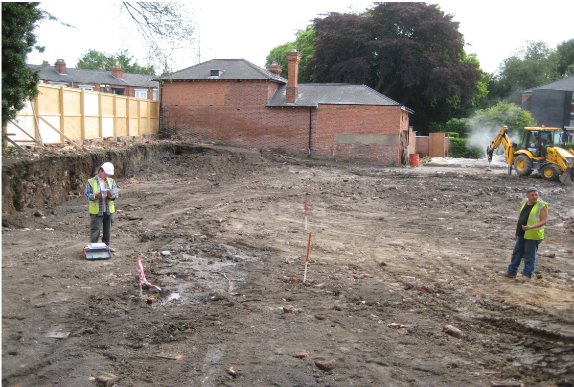
Plate 2 – General view of site
