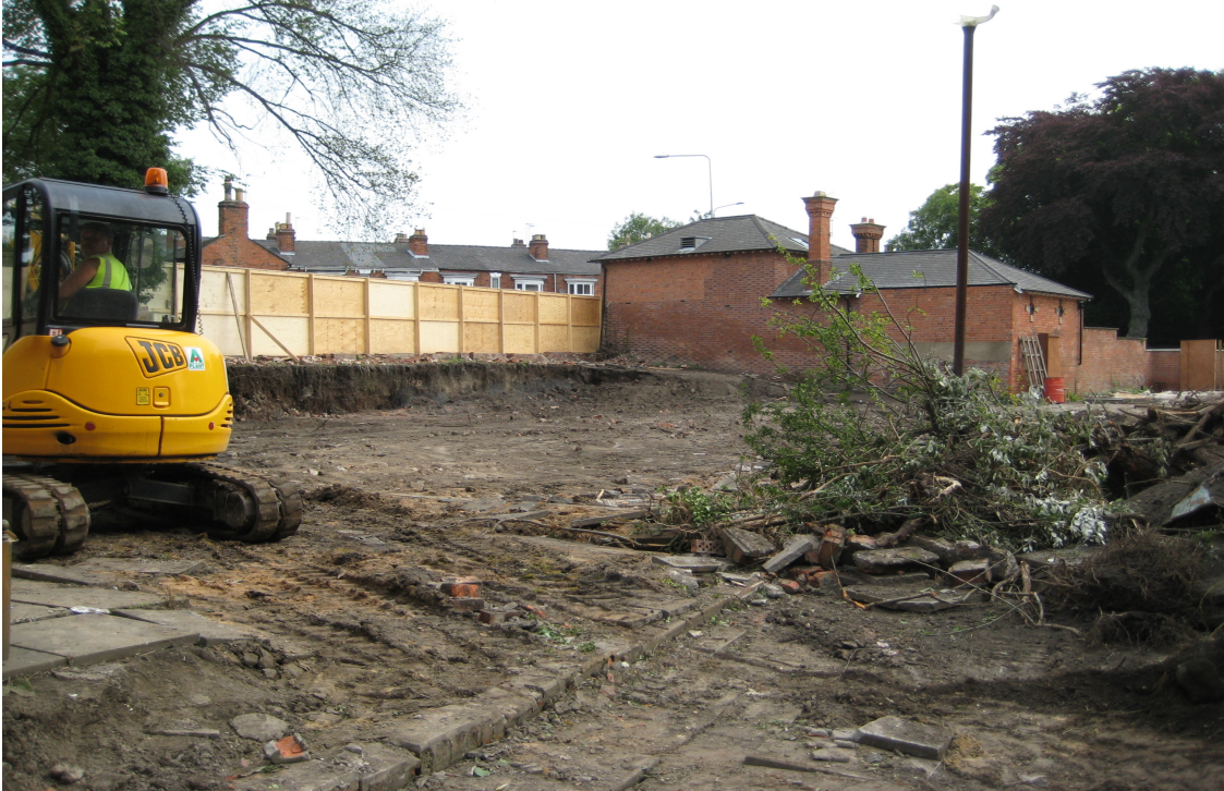
Plate 1 – General view of site
