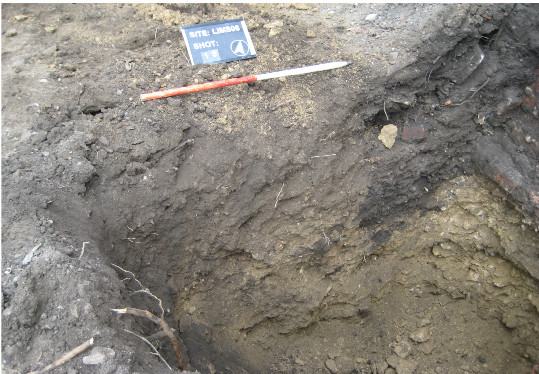
Plate 10 – Section 4: Excavation for underpinning of adjacent building
