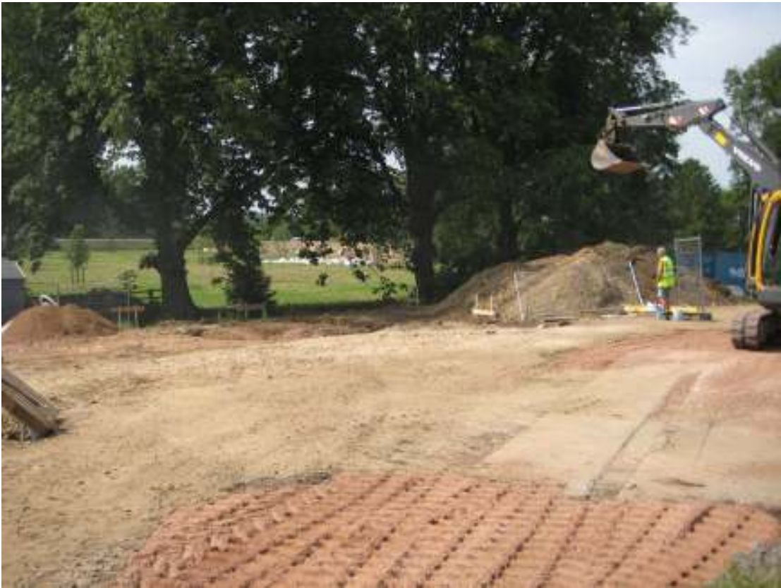
Plate 1 General Site View, looking west
