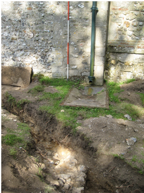
Plate 8 East facing view of wall (030) showing traces of a demolished wall in the western gable of the surviving church nave.
