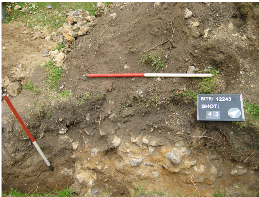
Plate 6 West facing view walls (030) and (035) after hand excavation of pipe trench (Section 8)
