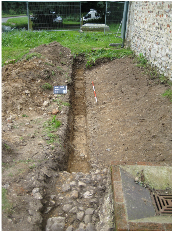
Plate 2 South facing view across Chancel excavation with wall (009) in the foreground
