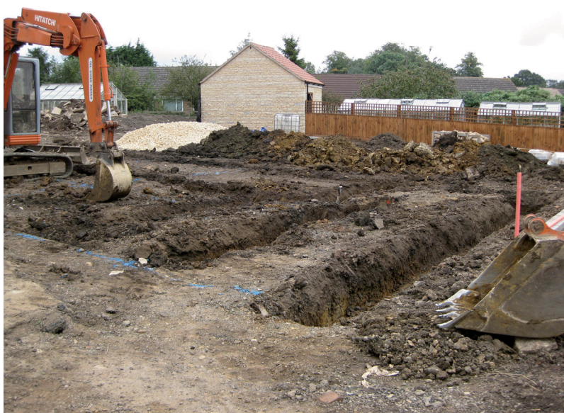
Plate 16 Watching Brief. General shot of groundworks in progress looking northeast
