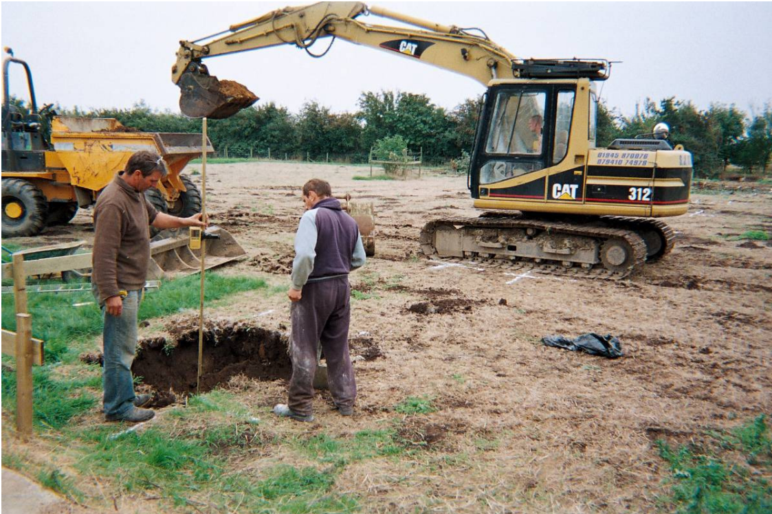
Plate 3 Excavation of Stanchion (Section 1) looking south-east
