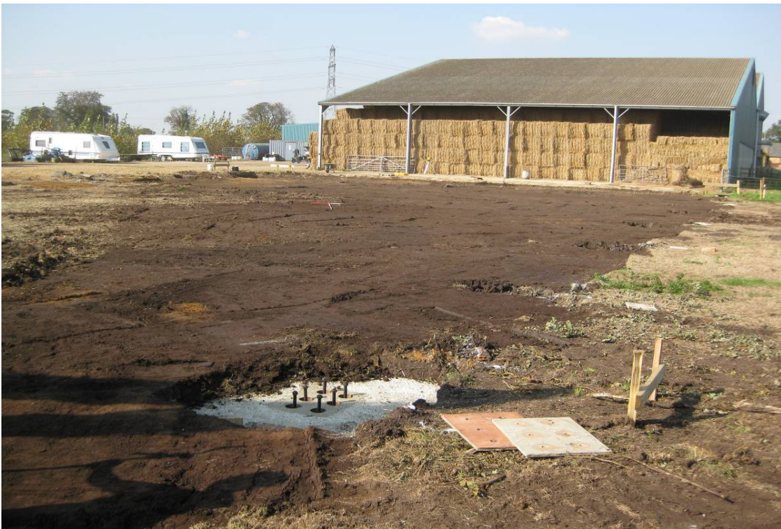
Plate 8 Site reduction looking north-west
