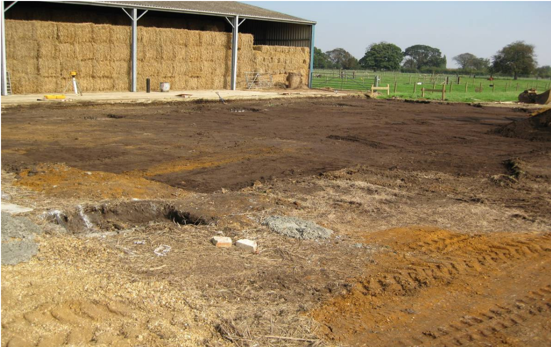
Plate 7 Site ground reduction looking north-east
