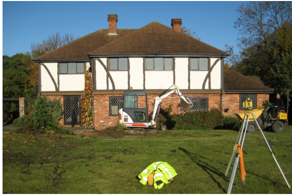
Plate 1 North facing view across site prior to the excavation of groundworks
