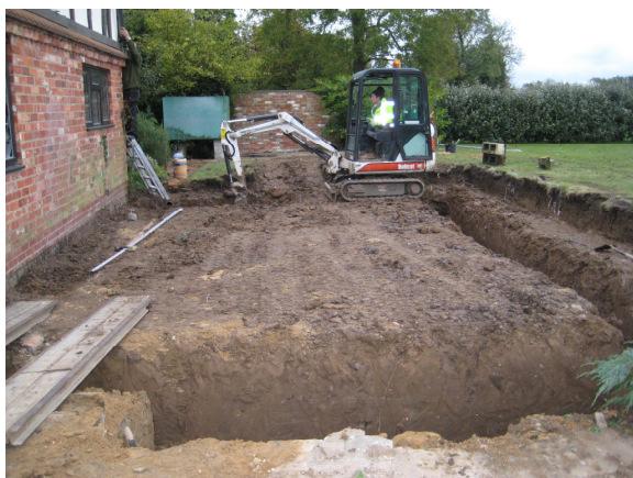
Plate 3 East facing view groundworks under excavation
