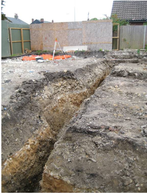
Plate 16 North facing view completed groundworks showing stone surfaces
