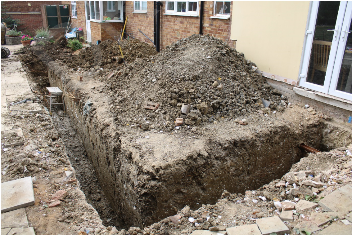
Plate 4. The completed footings, looking south
