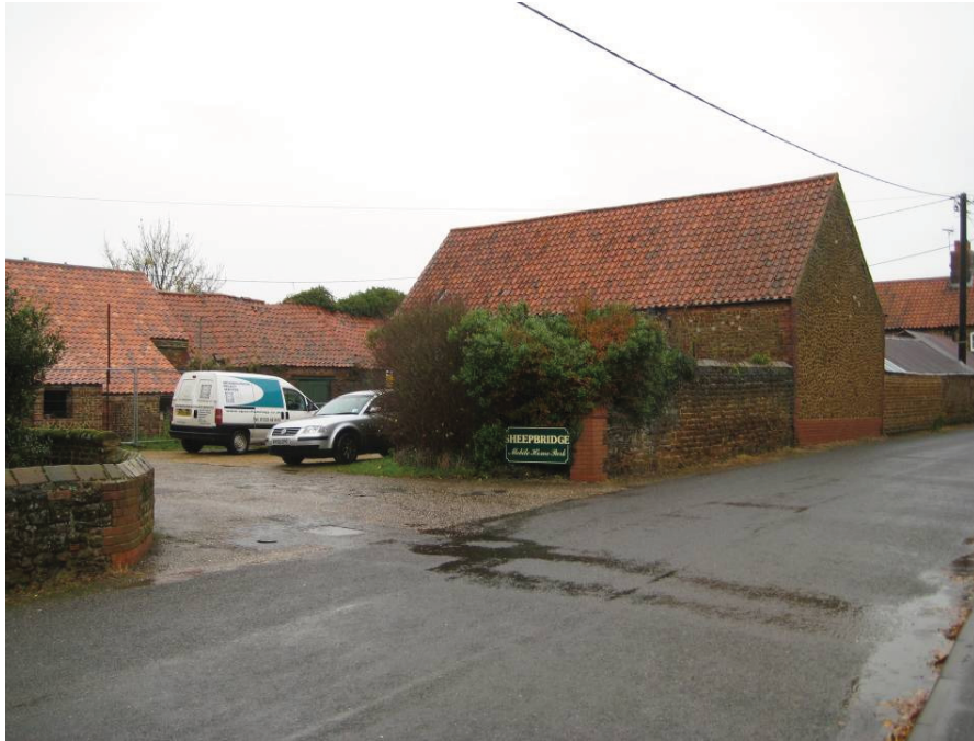
Plate 1 General view of buildings from Station Road, looking northeast
