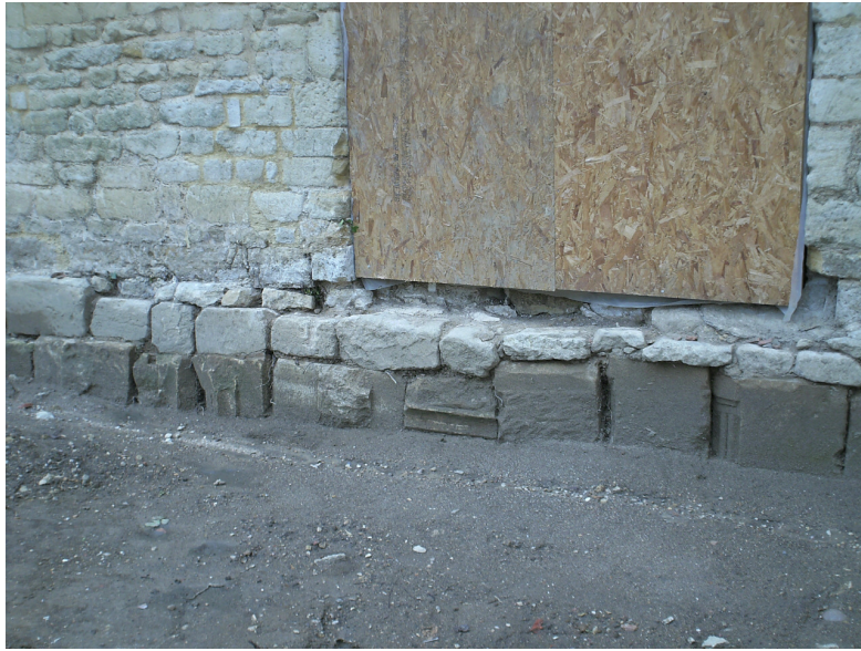
Plate 11 – View showing re-used masonry in foundations of barn, looking west
