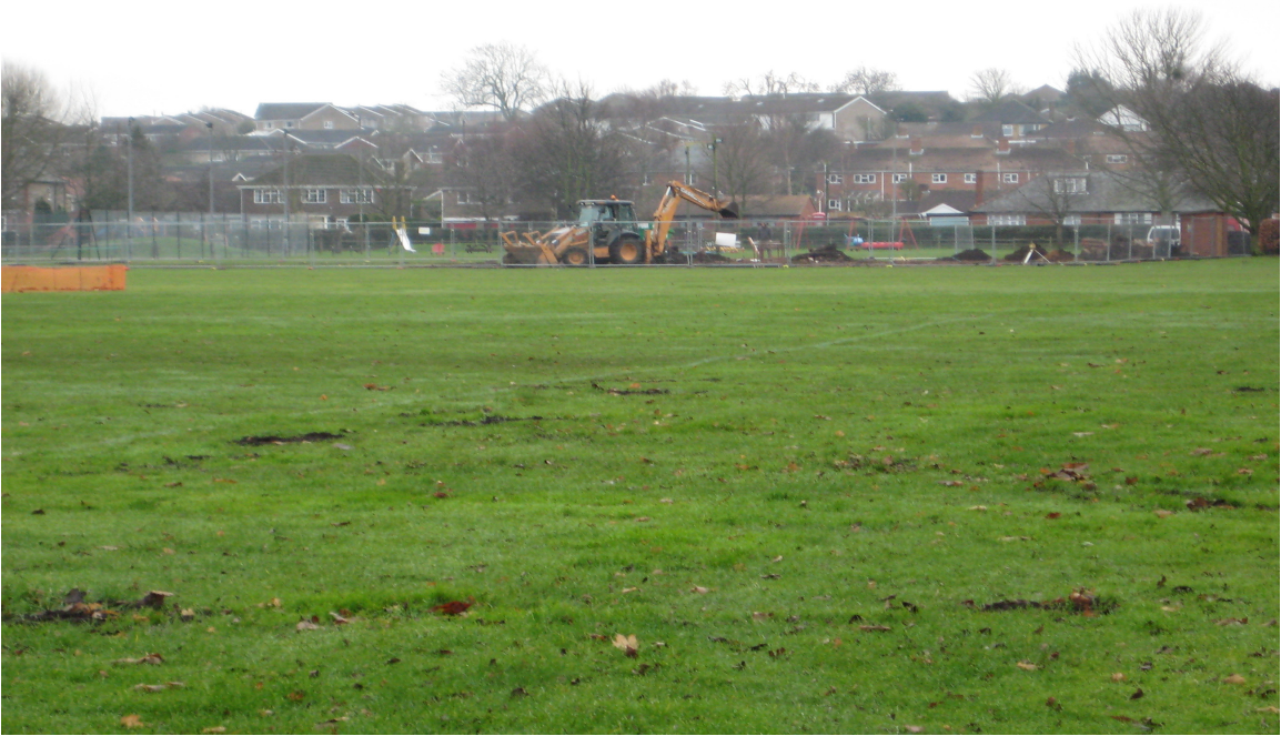
Plate 1: General site view looking south
