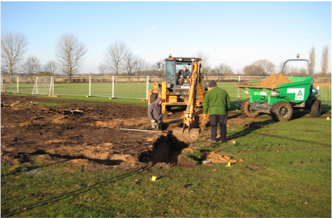
Plate 2: Foundation excavations looking north
