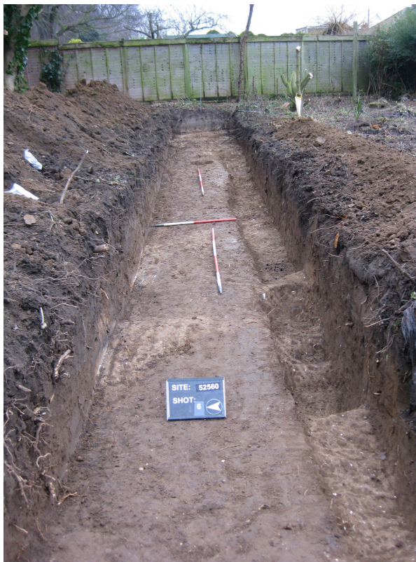
Plate 2 East facing view across excavation
