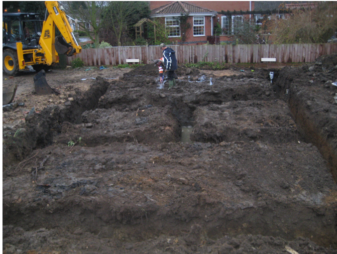
Plate 1 East facing view completed groundworks
