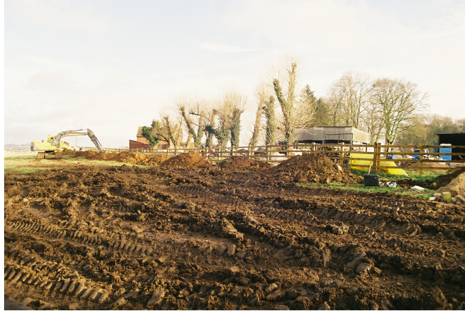
Plate 1 – General view of the area of works, looking northeast
