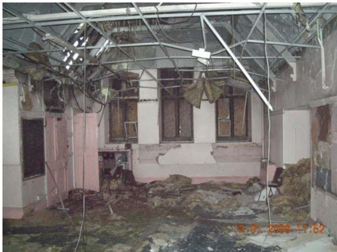
Plate 21 School room, looking southeast
