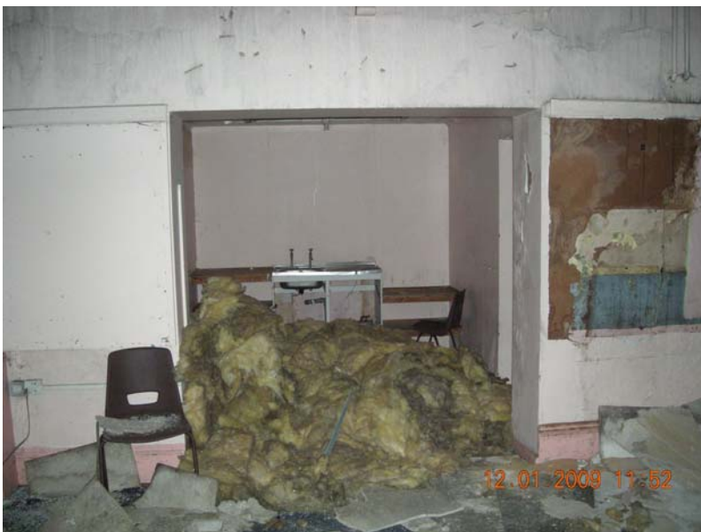
Plate 24 Inserted opening in school room east wall, looking west
