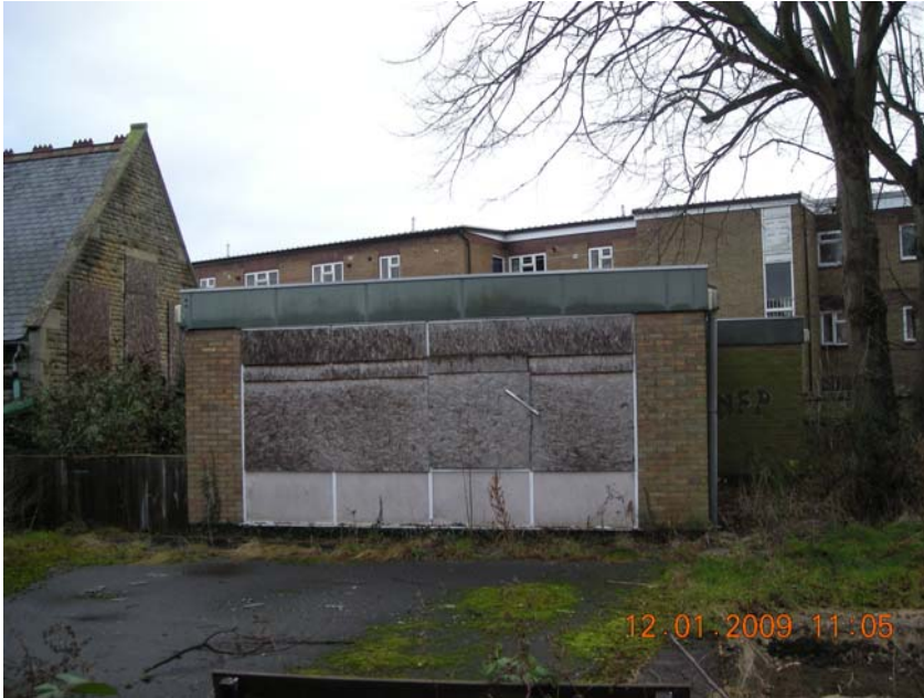
Plate 34 Extensions to southeast, looking east
