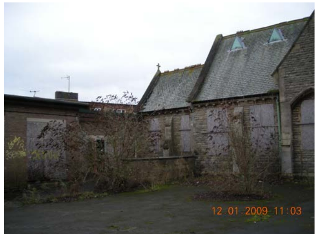
Plate 6 Northern elevation of chancel, showing cross finial, looking east
