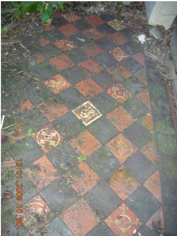
Plate 27 School house porch floor, looking north
