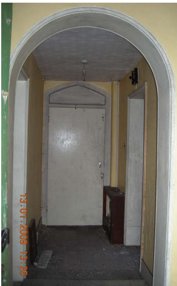
Plate 32 School house passage, looking east
