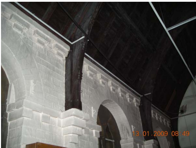
Plate 8 Detail of truss support timber in nave, looking north
