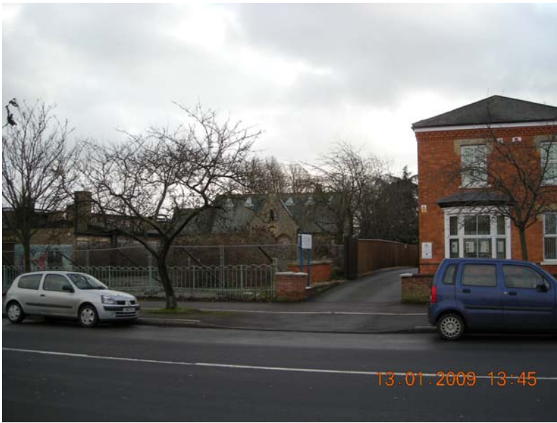
Plate 1 General view of school frontage, looking southeast
