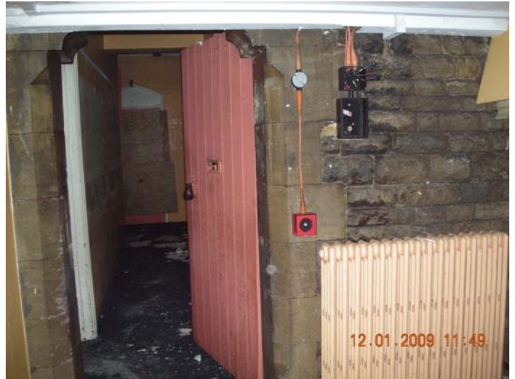
Plate 19 Original external door – door to corridor and view down corridor, looking west
