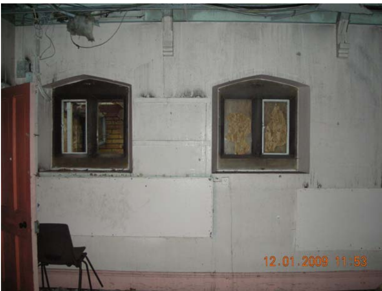
Plate 23 Windows in school room, looking east
